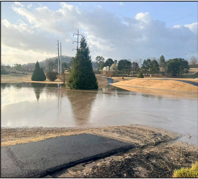
The Butternut Creek Golf Course experienced some flooding from the storm over the weekend. Photo/Facebook
